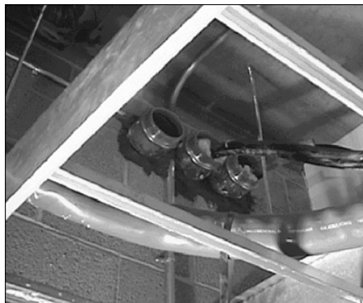
Figure A-36 Typical Firewall Penetration
