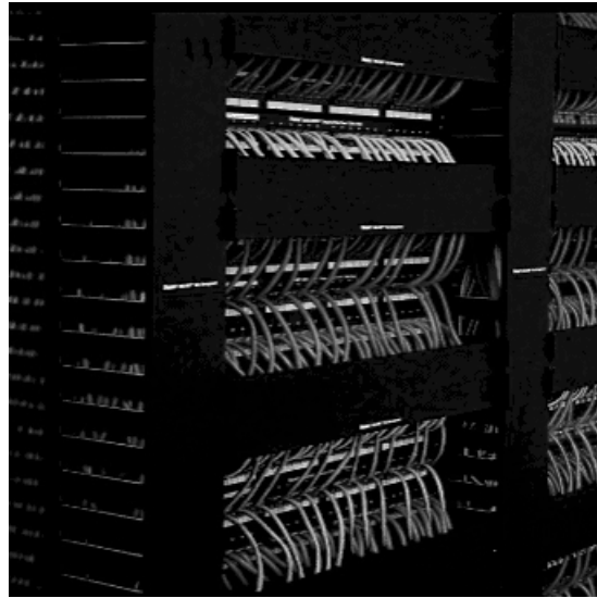
Figure A-8 Panduit Rack-Mounted Vertical and Horizontal Cable Management System
