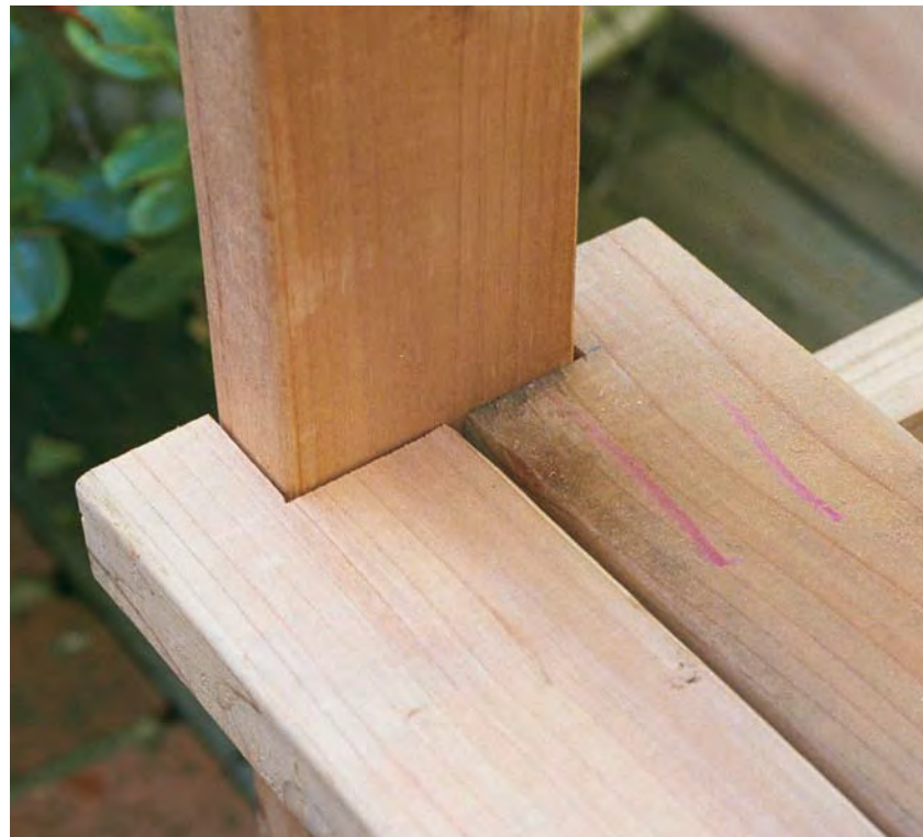
Overhang the edge of the lower shelf. Cut notches from each end of the front two boards to fit around the front legs.
