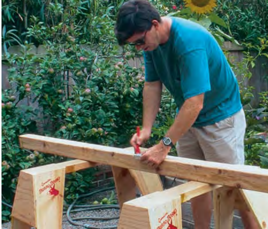
Measure, mark, and cut the side posts. You'll need only one 8-ft.-long 4x4 post for each bed because you'll cut it into four equal pieces, one for each corner (left). Attach three 8-ft.-long 2x6s to the corner posts with nails (right).
