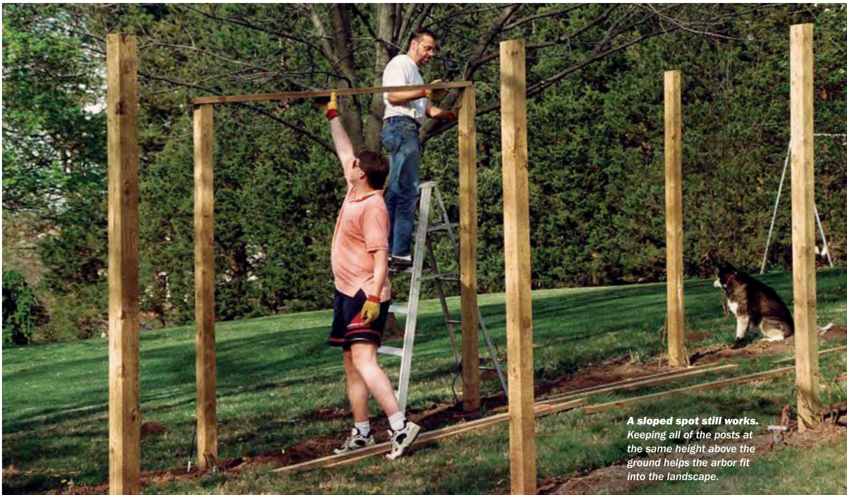
Let a machine do the work for you. With the help of a rented power auger, set the posts in holes 2 ft. deep. A post-hole digger would also get the job done, but more slowly.
