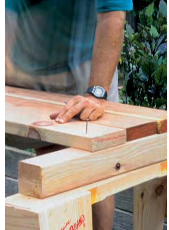
Measure, mark, and cut the side posts. You'll need only one 8-ft.-long 4x4 post for each bed because you'll cut it into four equal pieces, one for each corner (left). Attach three 8-ft.-long 2x6s to the corner posts with nails (right).
