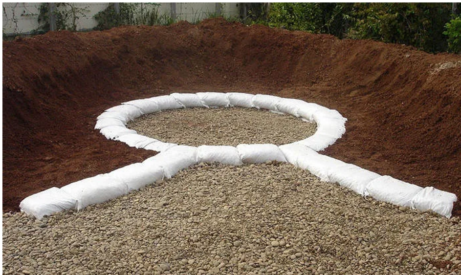
Earthbag dome foundation © Owen Geiger
